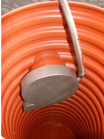
Fig. 6.11 Flow control chamber
